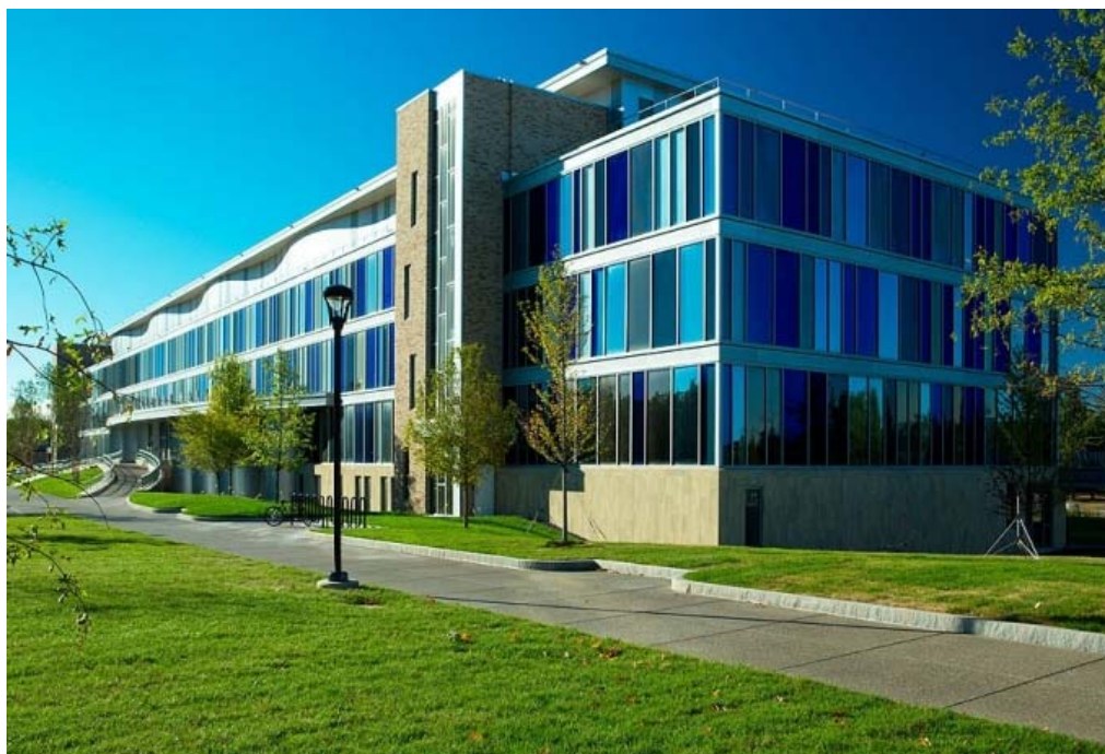
Through a NYSERDA-supported initiative, Kapoor Hall is projected to be 29-percent more energy efficient than required by the New York State energy code. Photo: DOUGLAS LEVERE
